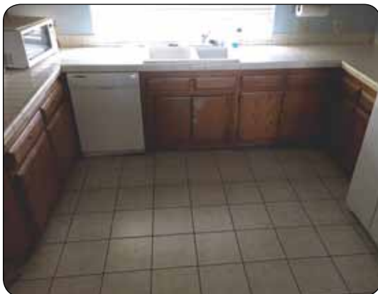
Before kitchen remodel
