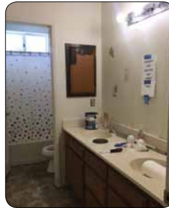
Before bathroom remodel
